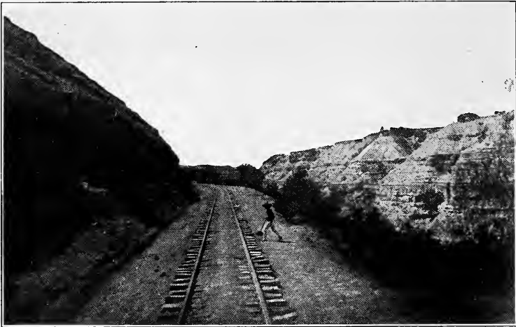
NOCHISTONGO CUT, BUILT BY THE AZTECS TO DRAIN THE VALLEY OF MEXICO.
